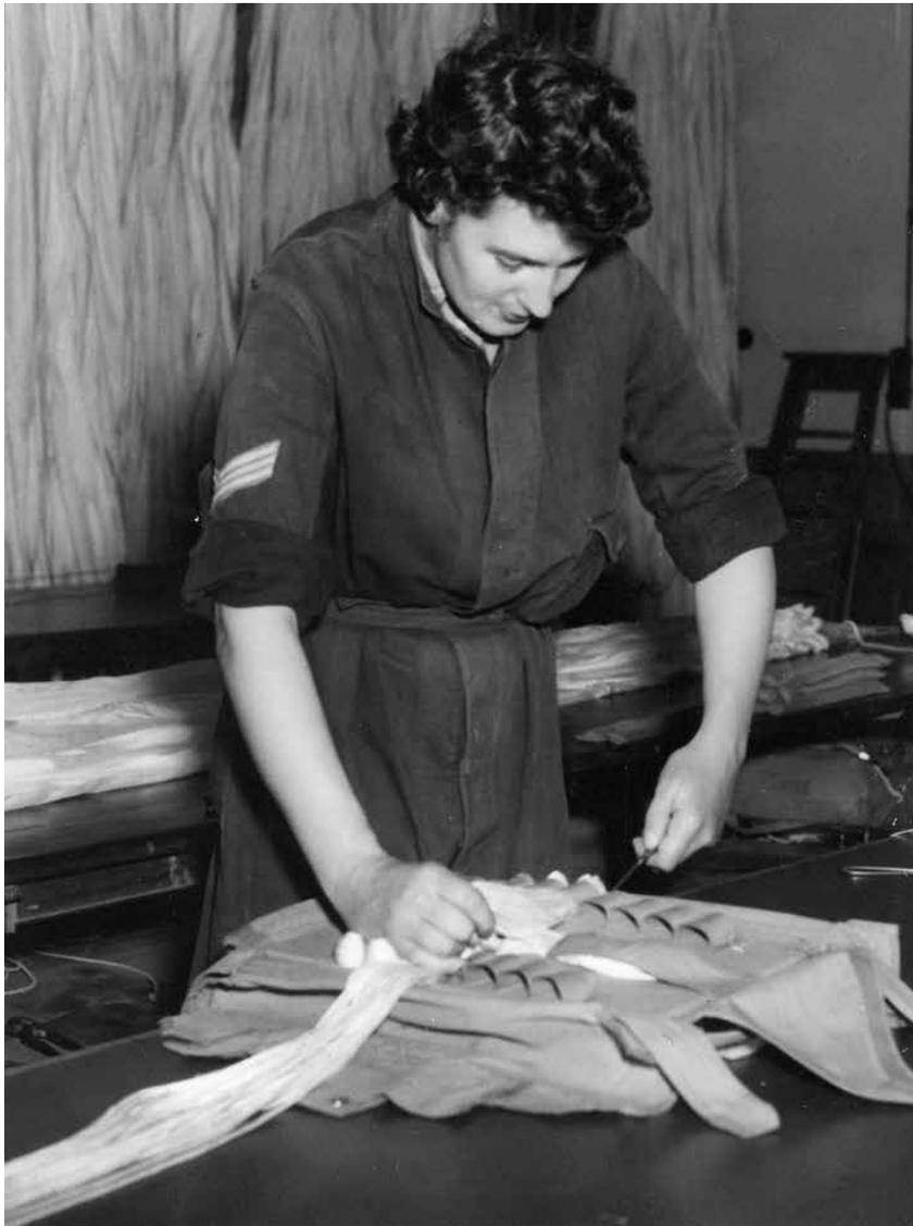
1942: packing rigging lines for a parachute (State Library of Victoria)
