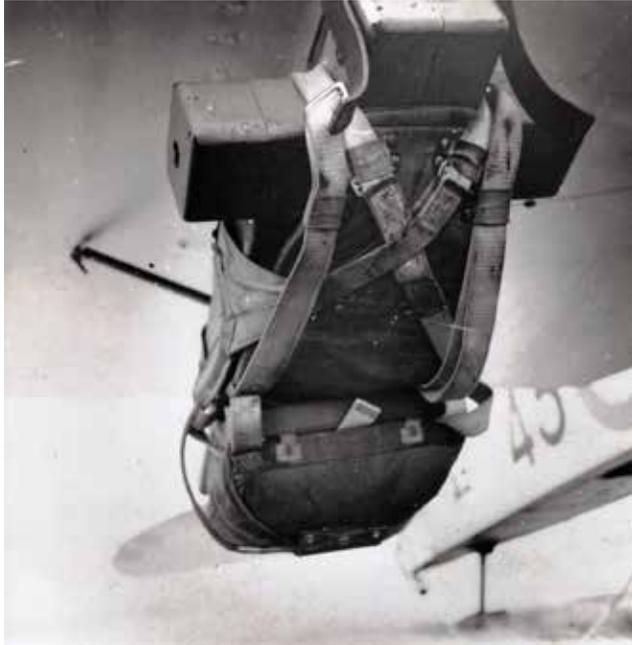
1926: wooden torso dummy for parachute testing mounted under the wing of a D.H.9 aircraft (RAAF Museum)
