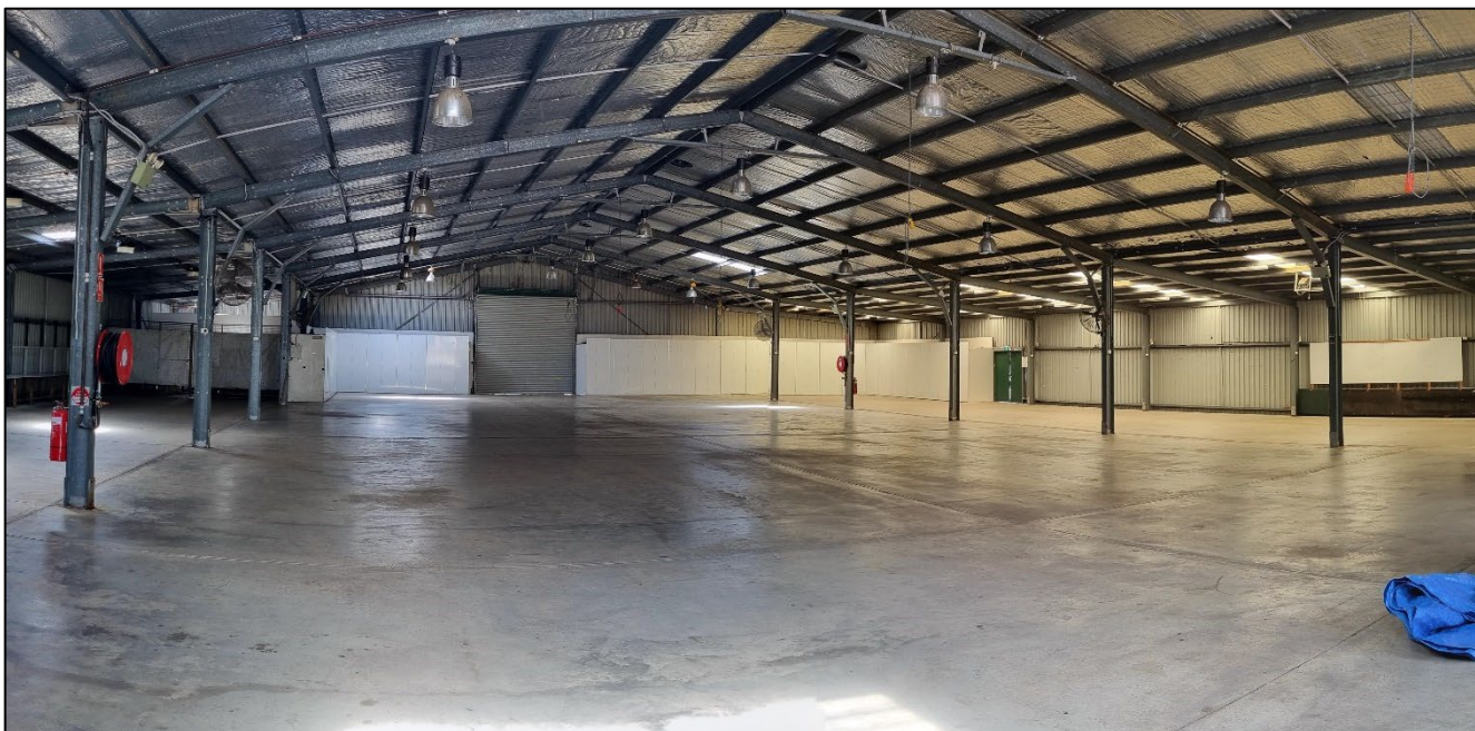
Interior of the huge pavilion.
